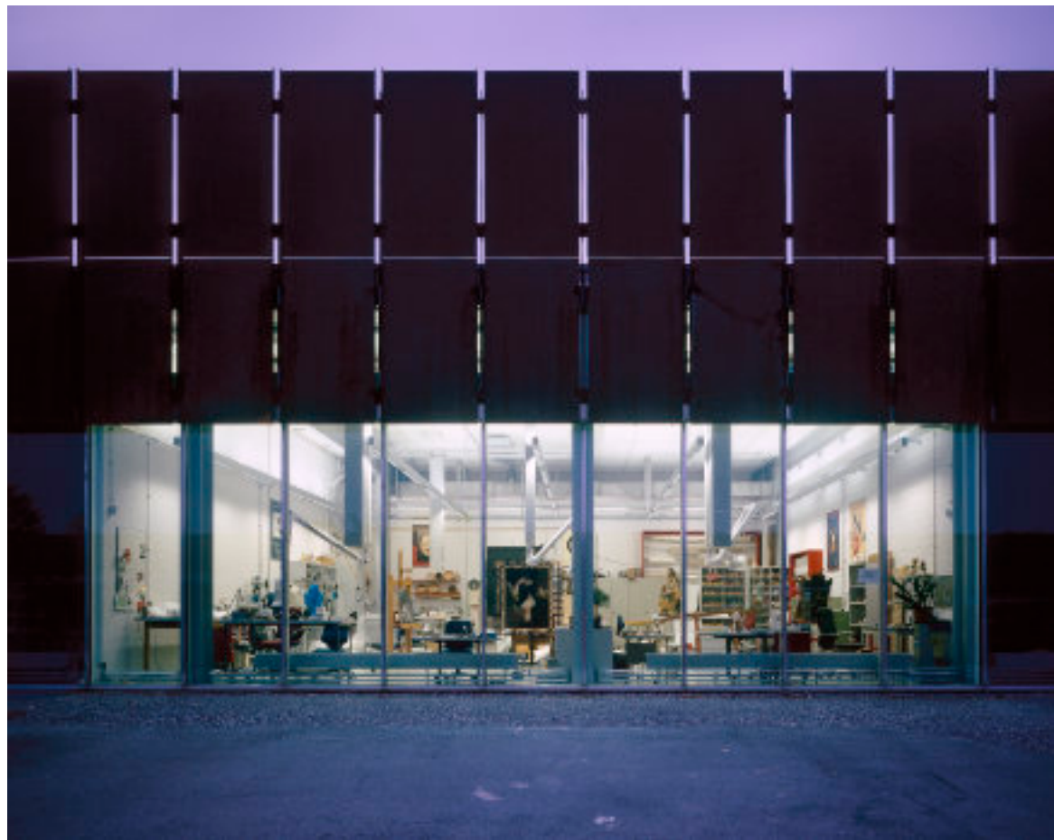
Images: Façade to the courtyard, slit of light in the outer façade, cultural goods store Plans: floor plan ground floor and cross-section
