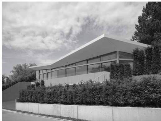
Pavilion House in Zumikon
